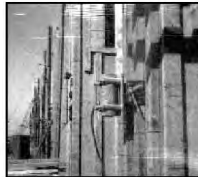
US-900 with wooden form clamp on column
