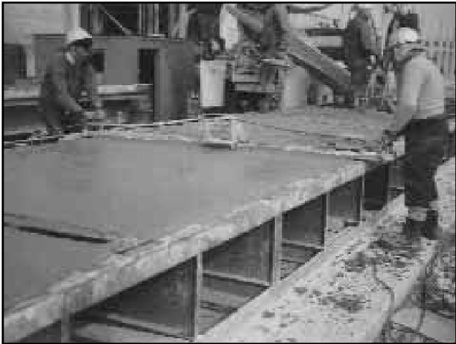
Model 2P-800 on 8' screed, made from a 6" channel iron with adjustable rods to minimize the bowing of the screed.
