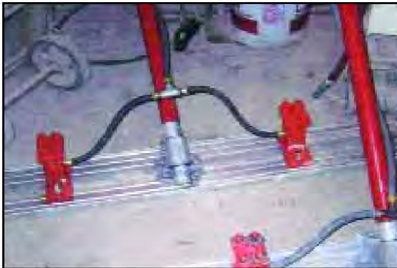
Screed with Model 50-1-1/4 pneumatic piston vibrator
