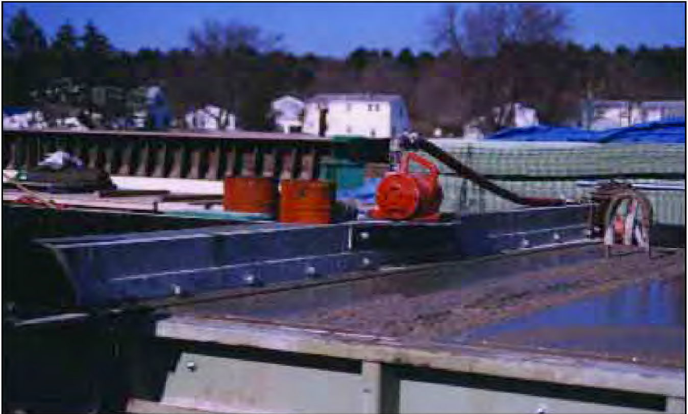
Model CCF-5000 Silent Pneumatic Vibrator on 10 ft. screed.
