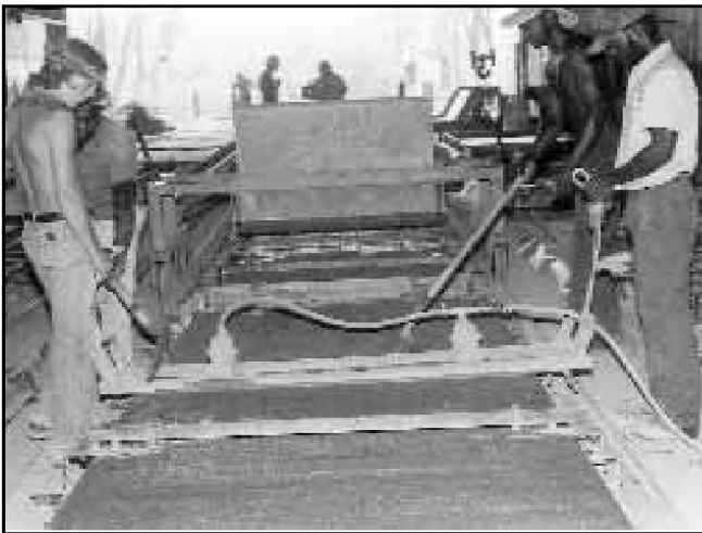
BVS-510FS Turbine Vibrator on 4" screed, made from 4" channel iron.
