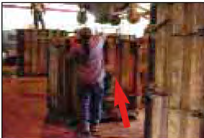
Two Model SVRLS pneumatic vibrators on lug brackets were mounted diametrically opposite on this box form.
