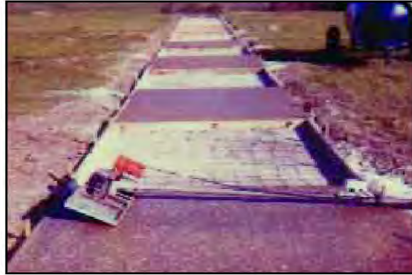
Finished sidewalk after it is washed.
