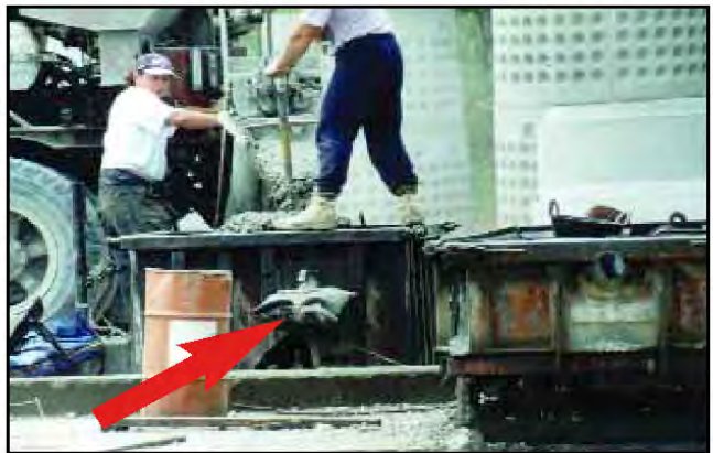
US-1600 with wedge on culvert form. (Notice a rubber sheet covers vibrator and protects it from concrete spill.)
