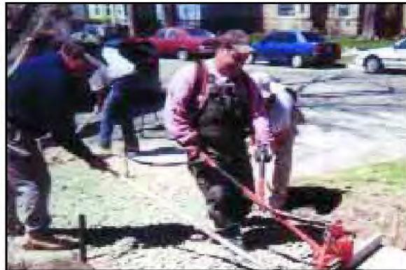
Screed using a 2 x 4 and a pneumatic VS-350 vibrator
