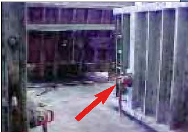
Two Model SVRLS pneumatic vibrators on lug brackets were mounted diametrically opposite on this box form.
