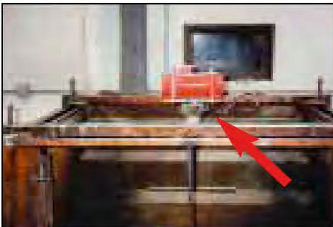
One Model 2P-200 115 Volt vibrator handles complete step form. 2P-200 attached to adapter plate & shoe bracket welded to form stiffeners (page 8).
